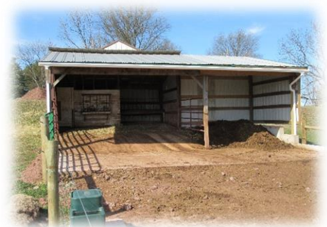
Example of a roofed solid manure stacking area
