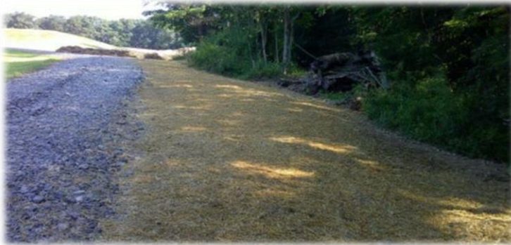
Temporary stabilization with straw
