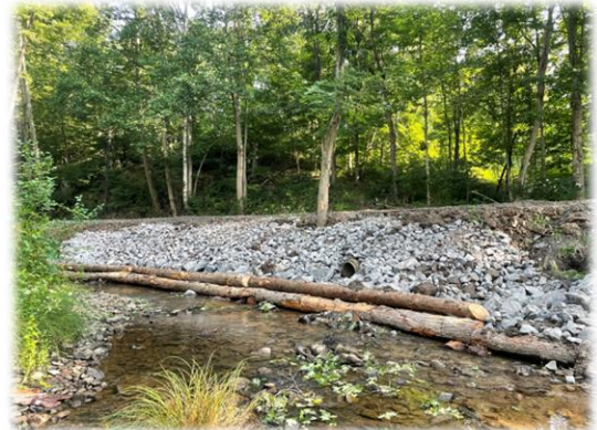
Mt. Pleasant Road streambank stabilization project
