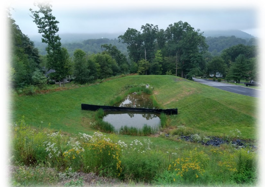
Rockville Estates Stormwater Infiltration Basin
