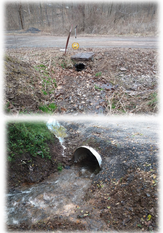
Reward Road– Phase 3 Greenwood Township Culvert Project
