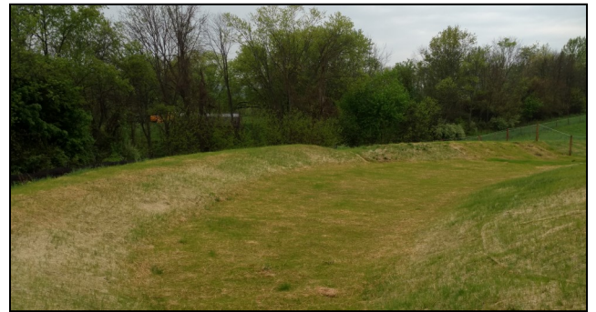
The new infiltration basin for Old Mill Estates in Shermansdale, Perry County.
