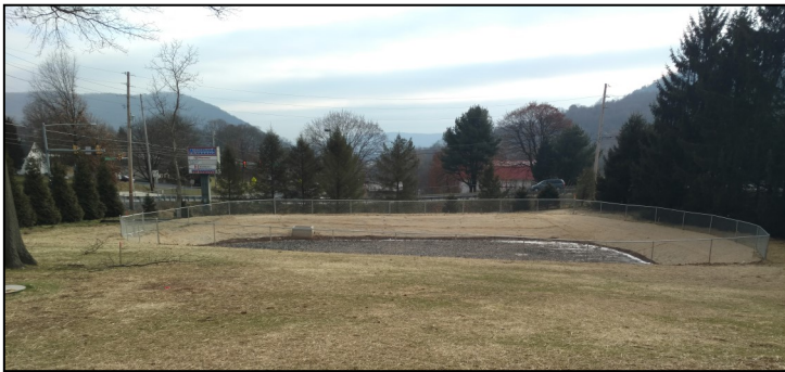
The new infiltration basin for the Dollar General in Duncannon, Perry County.
