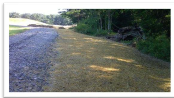
Temporary Stabilization with Straw
