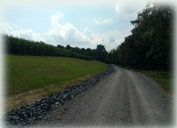
Bank stabilization project completed on Reward Road in Greenwood Township.
