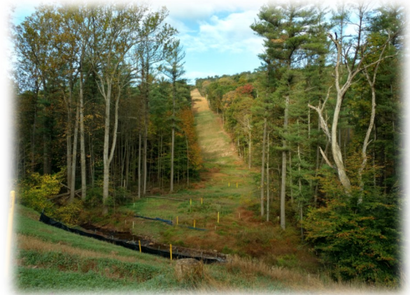
Sunoco Pipeline Vegetative Stabilization.
