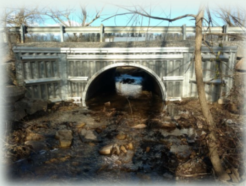
New stream crossing structure installed on Timber Road in Juniata Township.
