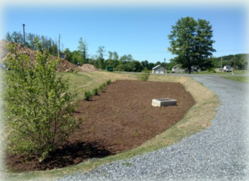
Constructed Rain Garden at Bible Baptist Church.
