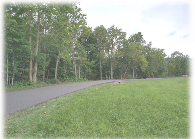
New DSA and culvert installed on Mt. Pleasant Road Jackson Township
