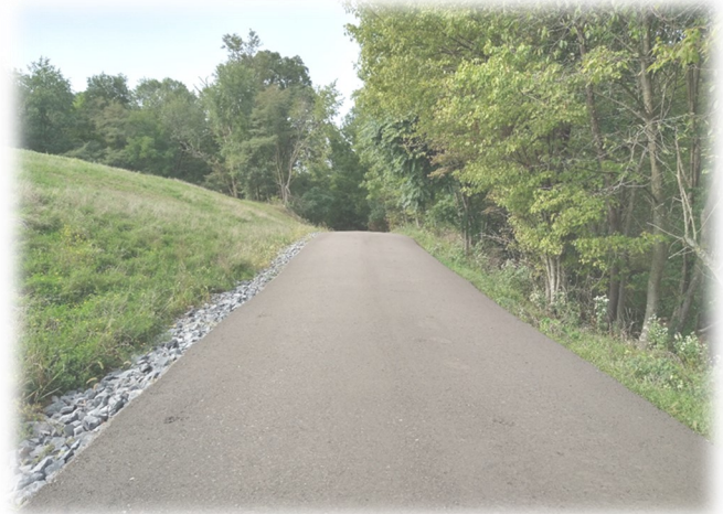
Newly placed DSA on Reward Road Greenwood Township
