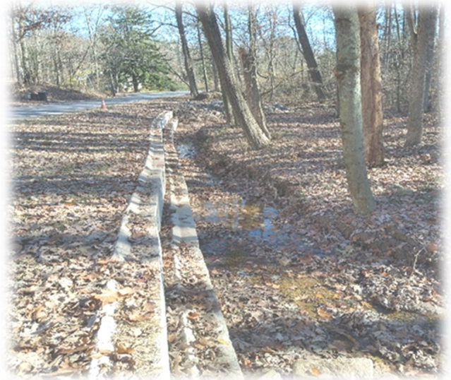
Meadow Grove Road Buffalo Township LVR Project
